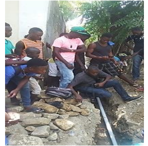
Figure 4: Connection to the main pipeline
