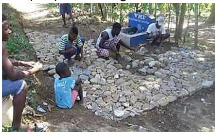
Figure 5: Pavement construction by the kiosk
